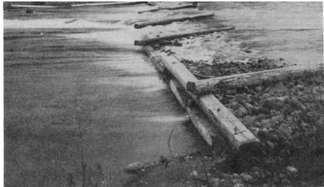
Dynamited crib dam at the foot of Lake Cle Elum. It had been built by opposing interests with Granger's timbers on, Granger's land. He had been denied the privilege to thus store water years earlier. When the illegal stream obstruction stopped water flow for his canal, Granger sent Engineer Tiffany and a powder crew to remove the structure. The crew went to jail and Tiffany was assessed a $500 fine, but once again water flowed in the Sunnyside Canal.
